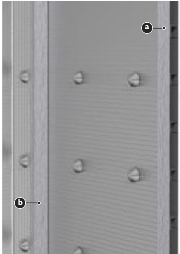
Detail of 60 minute load-bearing aluminium bulkhead
