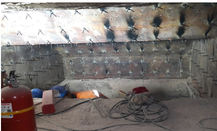
Figure 5: Welding studs for Pyro-Bloc Modules after marking with chalk lines
