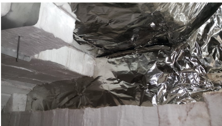
Figure 6: Stainless steel foil vapour barrier being installed
