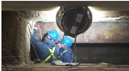
Figure 4: Measuring the distance for stud layout
