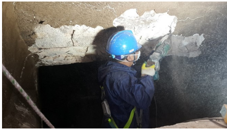
Figure 3: Demolishing original castable lining
